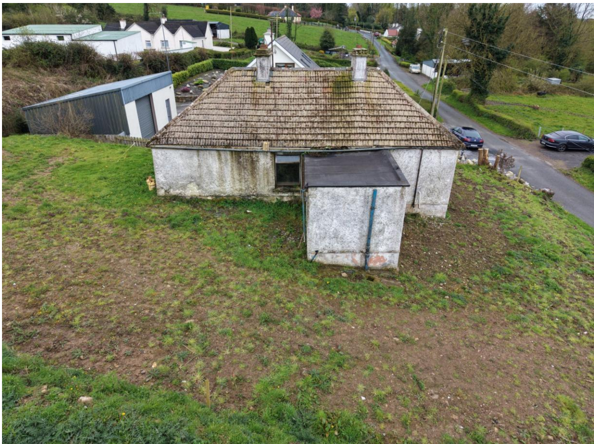
Derelict Residence, Ashbrook, Strokestown, Co. Roscommon
