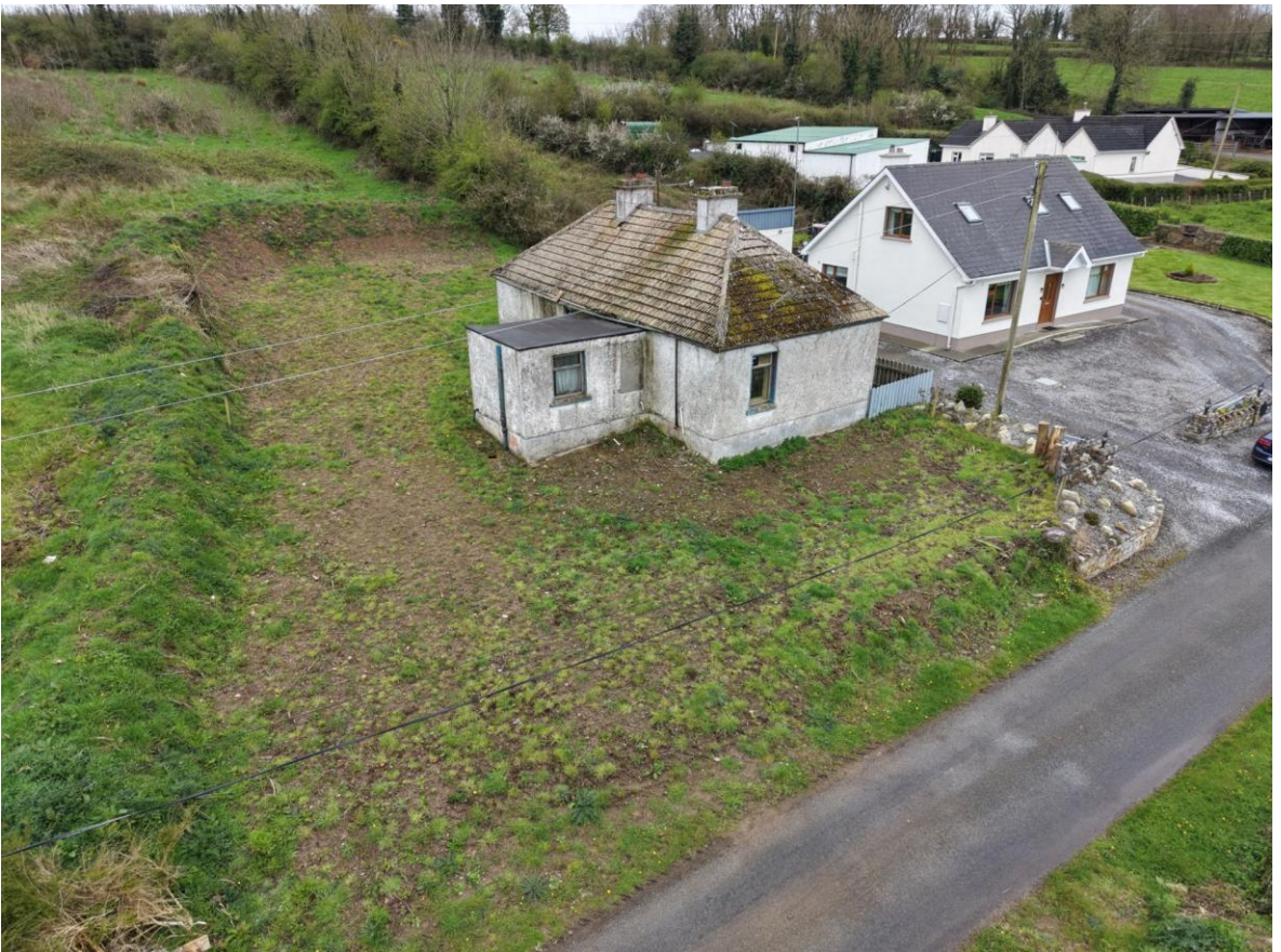
Derelict Residence, Ashbrook, Strokestown, Co. Roscommon
