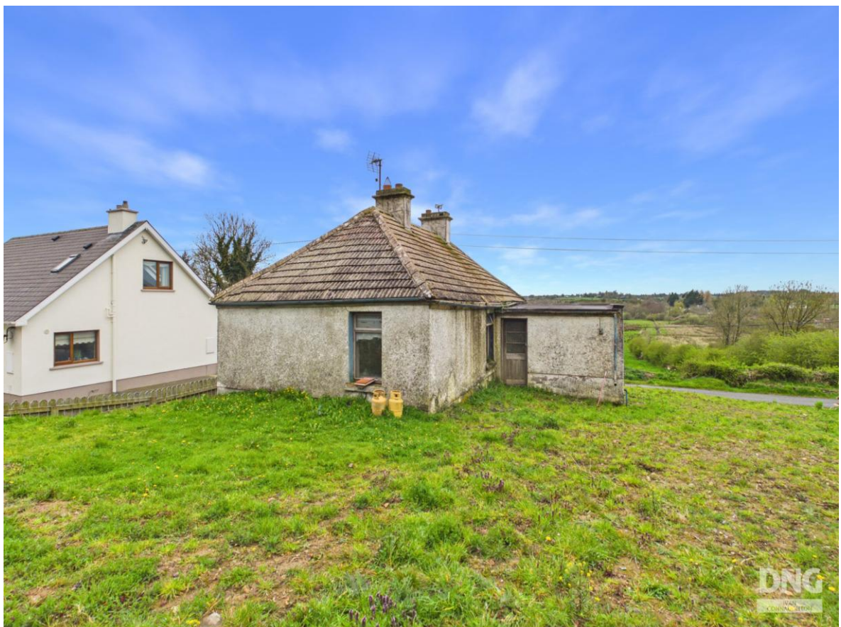
Derelict Residence, Ashbrook, Strokestown, Co. Roscommon
